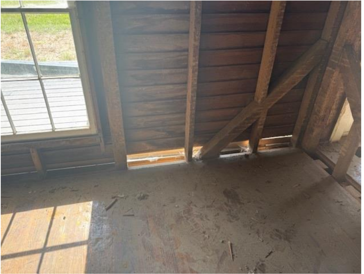
Figure 7. Missing siding exposing the inside of the structure to the elements (photo from Staff)
