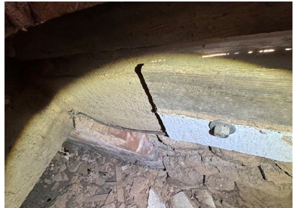
Photo 12: Brick Foundation Adjacent to Stone with Mortar Foundation
