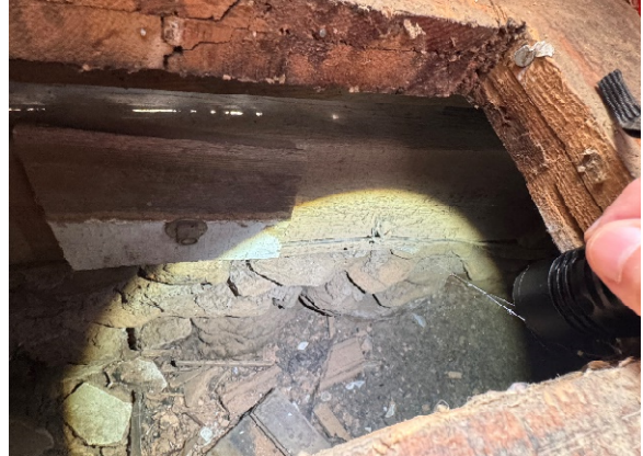
Photo 10: Stone with Mortar Foundation
