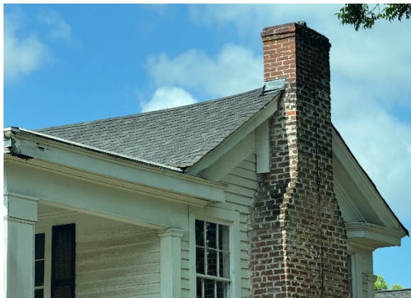
Photo 7: Differential Building Settlement
