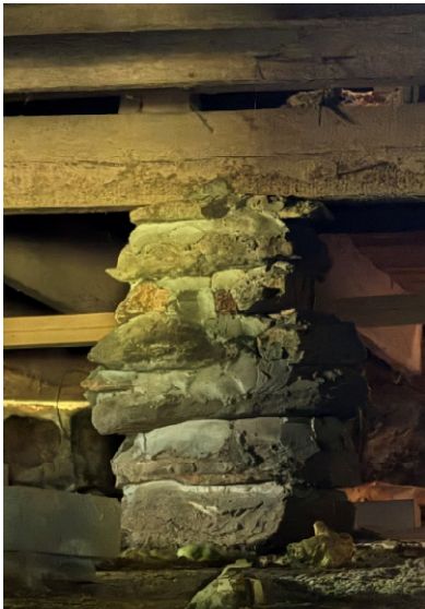
Photo 11: Stone with Mortar Foundation
