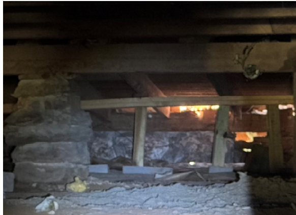
Photo 15: Retrofit Concrete Blocks Bearing on the Soil
