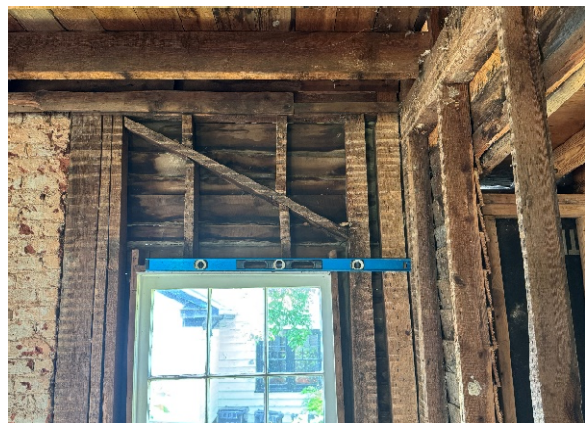
Photo 8: Differential Building Settlement
