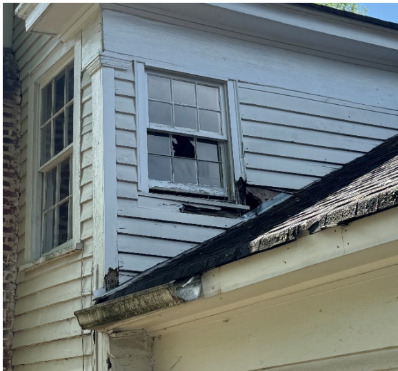
Photo 3: Rotten Siding
