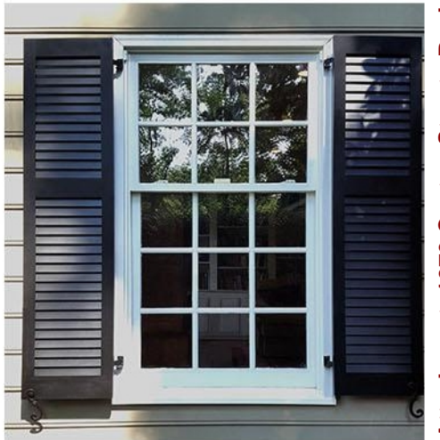
ALUM. CLAD WOOD WINDOWS W/ 5/8" MULLIONS & OPERABLE SYNTHETIC WOOD SHUTTERS, PAINT FINISH (SEE MUNTIN DETAIL - LEFT)
