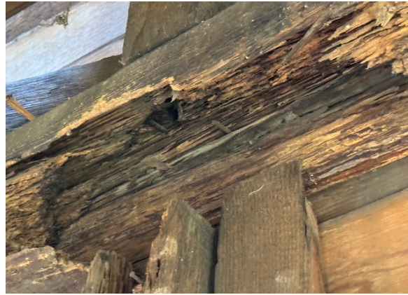
Photo 2: Rotten 4x8 Beams
